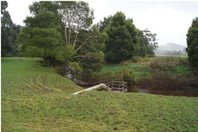
Wannon Water's Otway South water offtake on the Gellibrand River. Livestock have unimpeded access to the river at this point.
